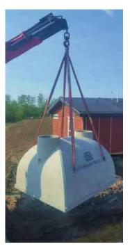
Our CSA certified septic and sewage holding tanks are tested for a burial of up to 3m. PCP tanks are constructed with 40 MPA - Type 50 concrete, as well as steel reinforcement to ensure strength and integrity.
